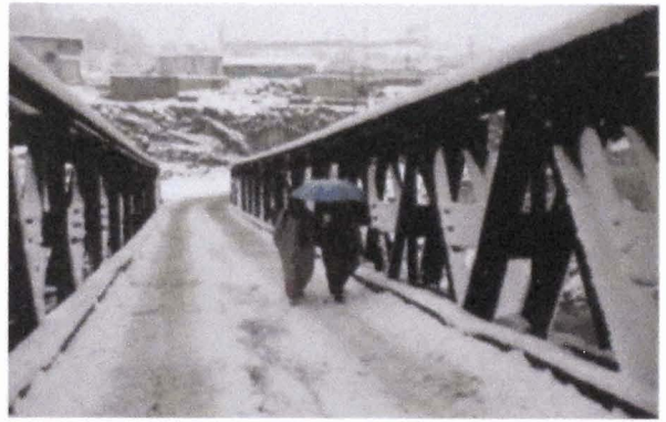
Iqbal Bridge over Suru River (1954, named after L/Nk Iqbal Singh).
